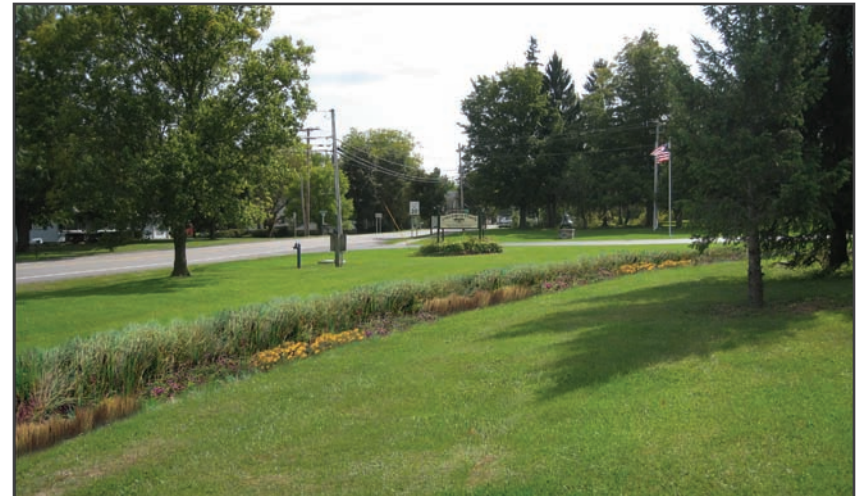
Drainage Swale After
