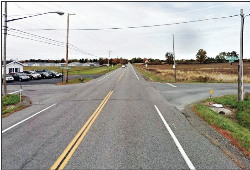
Looking North on Route 15A
