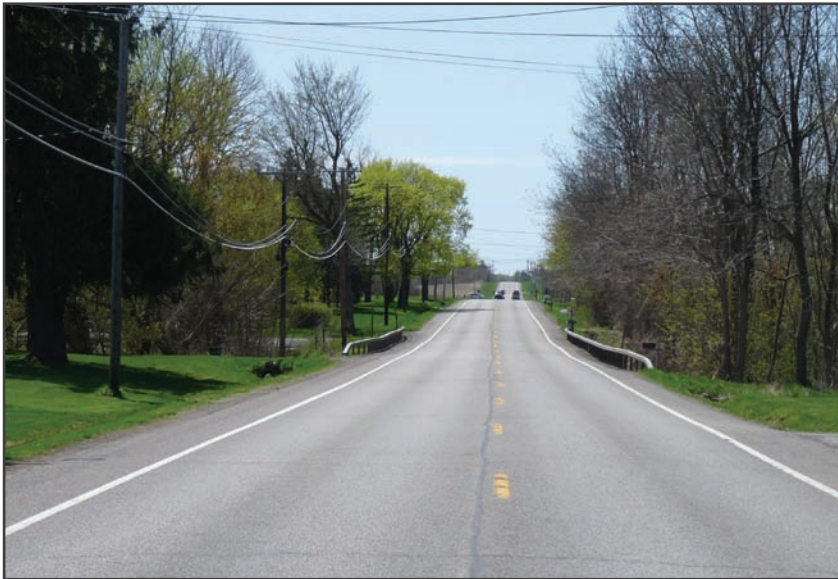
Spring Brook Bridge Before
