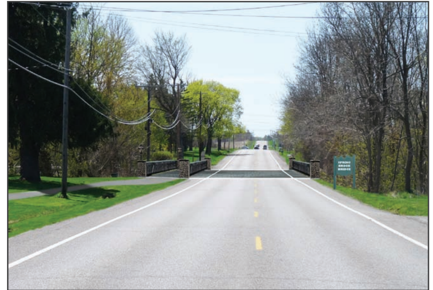
Spring Brook Bridge After
