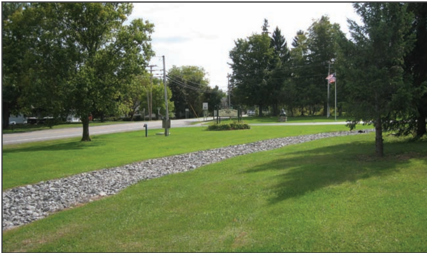
Drainage Swale Before
